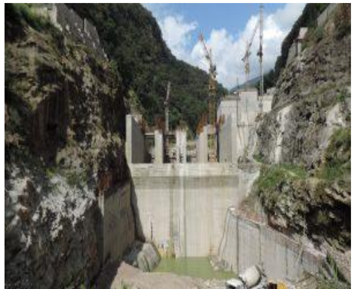
Dam from downstream
