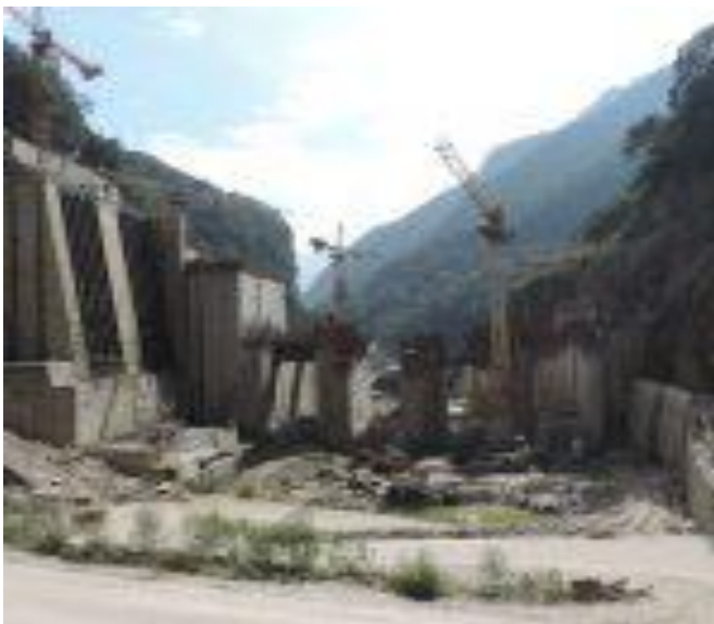
Source: MHPA website- Dam and intake from upstream
