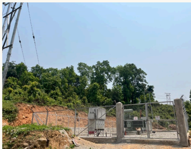
33/11kV, 2.5MVA Substation at Yoeseltse
